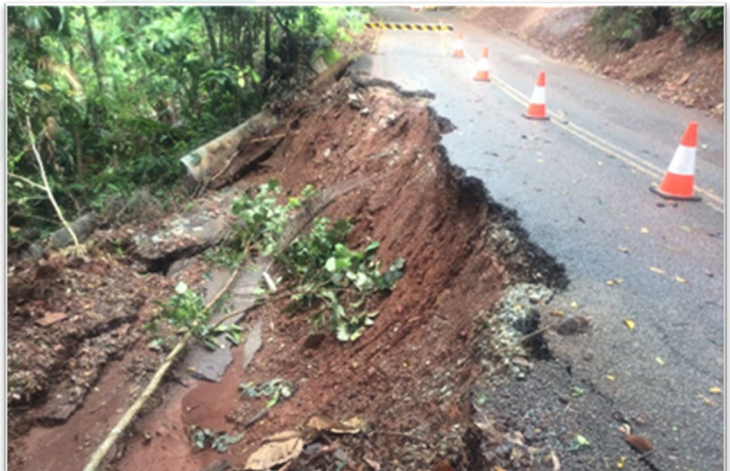
Road collapse caused by heavy rainfall
